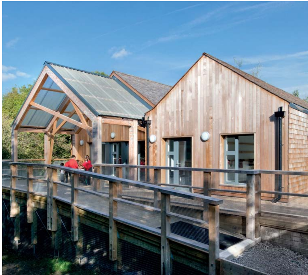
The building's construction makes use of natural and reclaimed materials, including straw bale insulation, timber off-cuts and even car tyres
